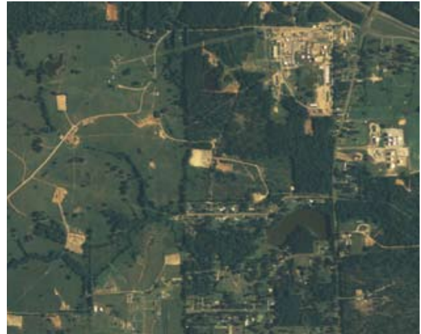
East Texas view in the Haynesville area including numerous well pads and facilities.
